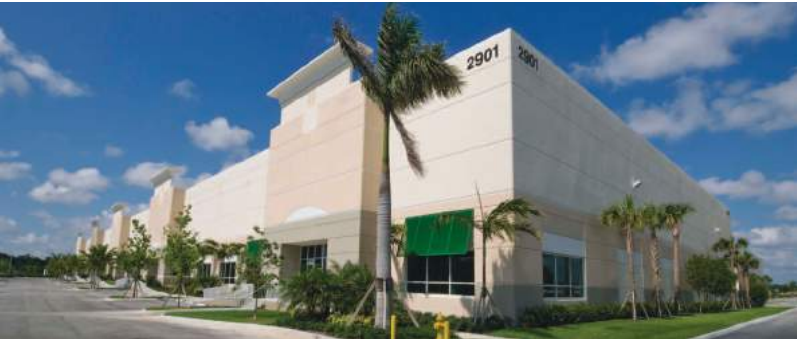
Photos from left to right – facing page: 6600 Port Road - Columbus, Ohio; Rickenbacker 936 - Columbus, Ohio; this page: Baylor Orthopedic & Spine Hospital - Arlington, Texas; Department of Defense BRAC 133 Office Complex - Alexandria, Virginia; Pompano Commerce Center - Pompano Beach, Florida
